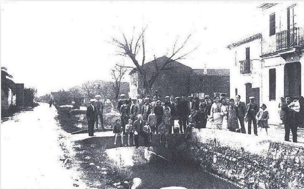
PHOTO 8. Building from 1911 at the intersection of Jesús Morante Borrás Avenue and Caminot Street.
