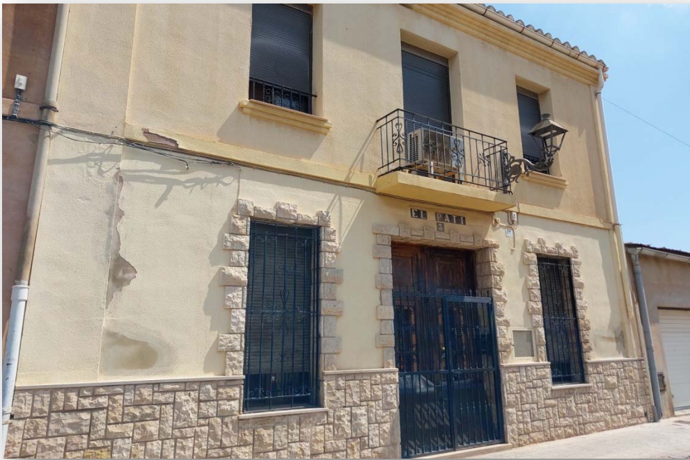
PHOTOS 5 and 6. House "El Pati"
