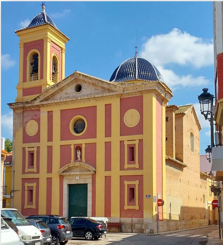
PHOTO 2. Church of Santa Ana
