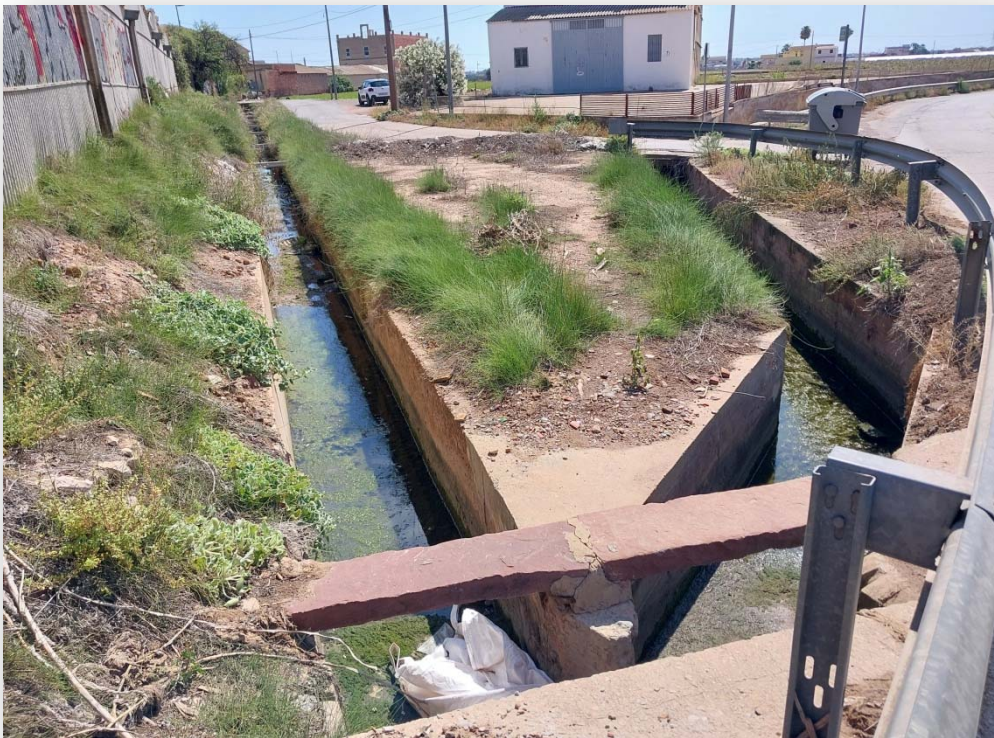
PHOTO 2. Bifurcation of the Tormos irrigation canal known as the Ferrús-Borbotó tongues.
